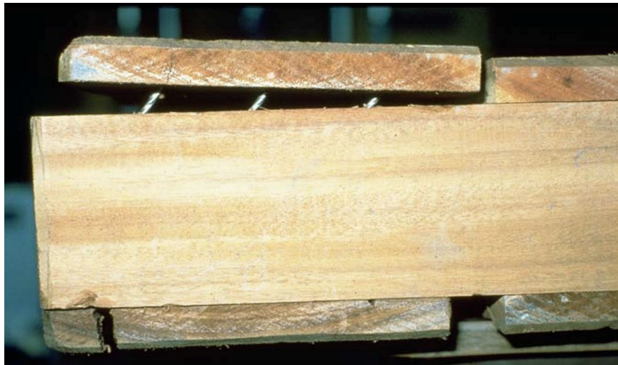
Figure 8. Showing fastener shearing causing pallet joint separation.
