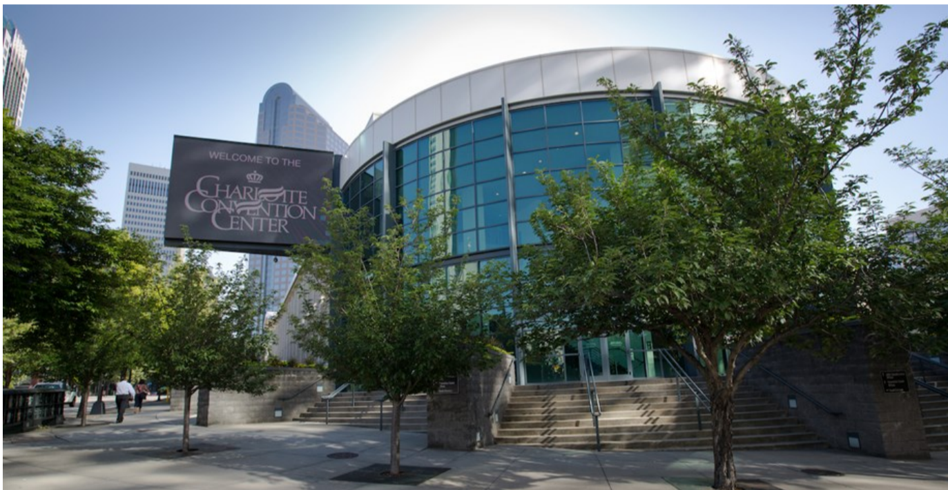
The Charlotte Convention Center is one of two venues in North Carolina that recently earned GBAC Star certification. Photo Credit:Charlotte Regional Visitors Authority
