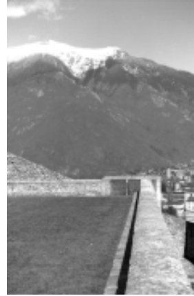
The castle renovation in the Ticino town of Bellinzona exhibits the architect's mastery of working modern building materials into a medieval context. This new castle courtyard has elements of sitecast concrete and concrete masonry units within the old existing stacked stone walls, which for the design of the villa expansion are a strong precedent for a parallel way of thinking and building.
