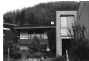
In a region where retaining wall construction is often the first critical act in the building process, the hillside towns of Gandria and Rovio are stacked insertions into the landscape.
