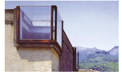
3.25 | Gipsoteca Canoviana, Carlo Scarpa, exterior window detail
