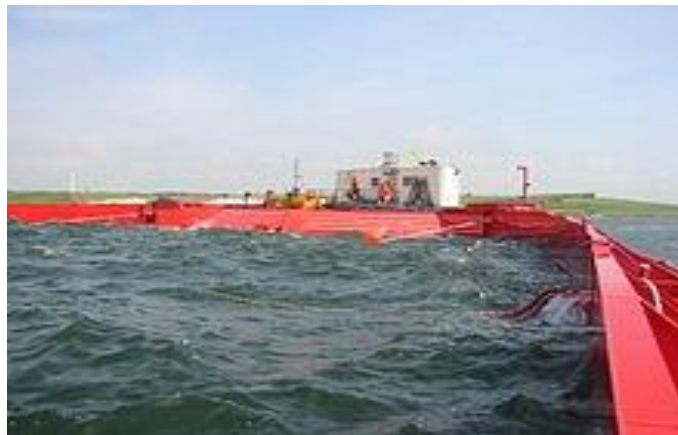
Figure 1-5 Overtopping device Wave Dragon prototype deployed in Denmark as proof of concept
