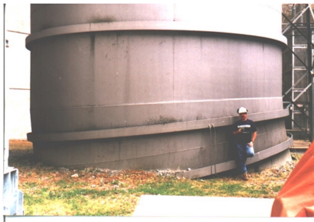
Figure 3-3. 26 ft Penstock at Smith Mountain Dam
