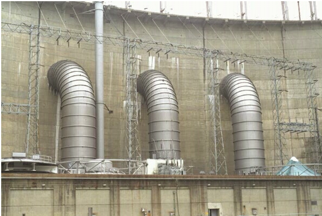
Figure 1-3. Smith Mountain Dam
