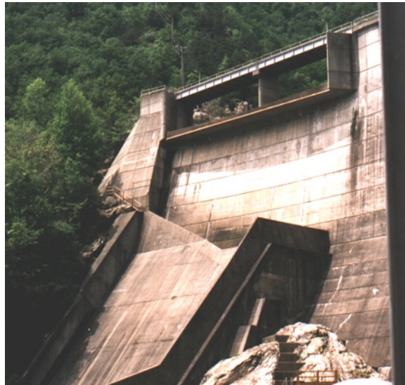
Figure 3-4. Left spillway at Smith Mountain Dam
