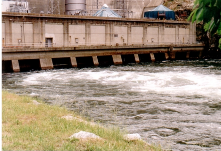
Figure 3-2. Tailrace of Smith Mountain Dam power
