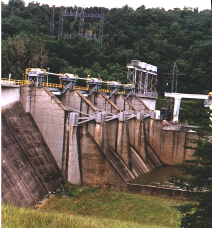
Figure 3-5. Leesville Dam and Spillway
