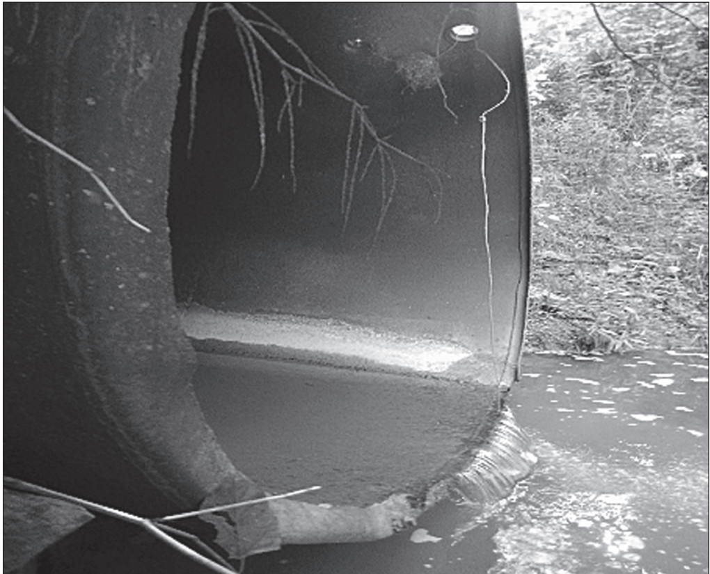
Figure 1. A perched road culvert at Hart Creek site 2.
