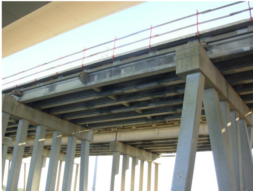
Figure 1 Deterioration in the Lesner Bridge (Alfailakawi et al., 2020)
