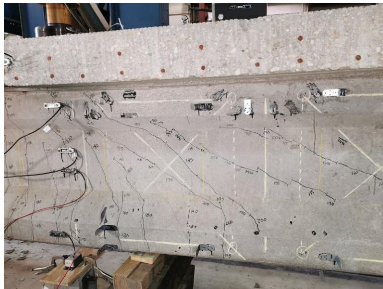
Figure 47 Cracking pattern for the first Lesner test (inland side)
