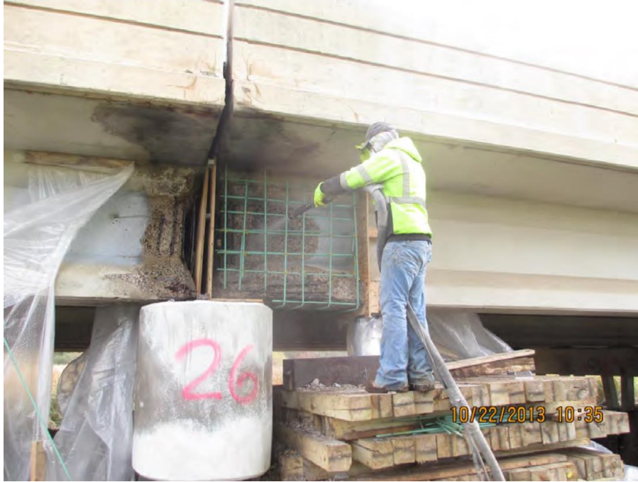
Figure 23 Rehabilitation technique used in Shield et al. (2018) (Shield et al., 2018)
