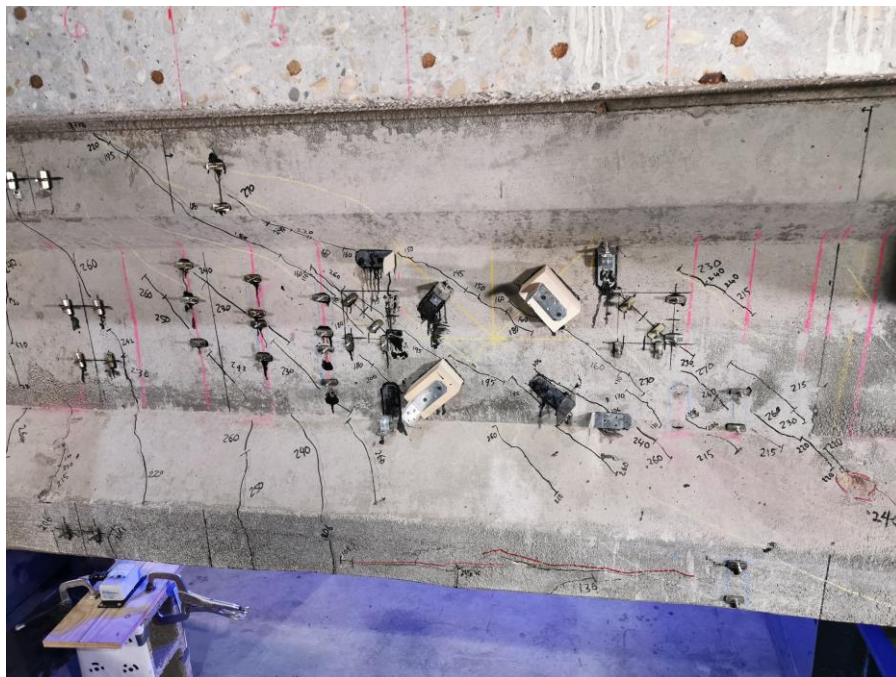
Figure 50 Cracking pattern for the second Lesner test
