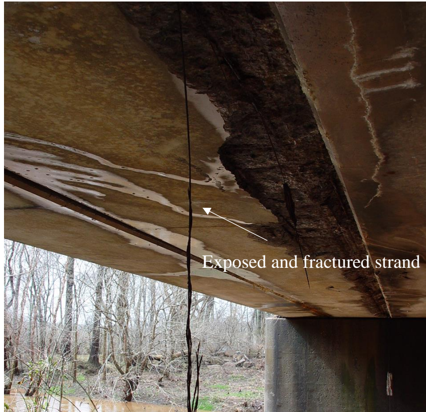
Figure 2 Deterioration in the Aden Bridge (Alfailakawi et al., 2020)
