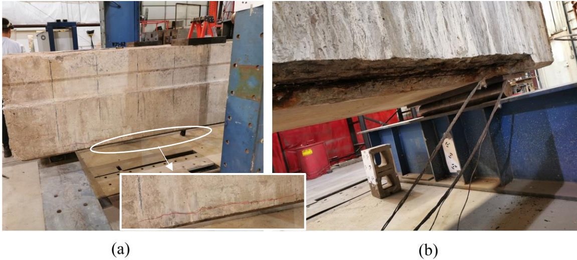
Figure 26 Aden girder end regions. (a) Less damaged end. (b) More damaged end with section loss and exposed strands
