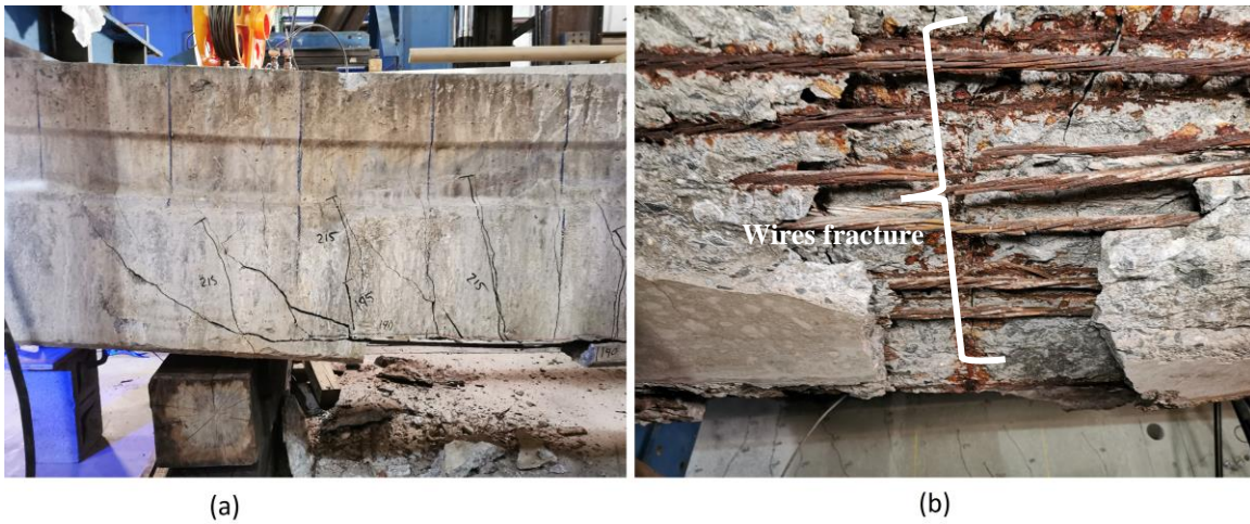
Figure 57 Failure mode for the second Aden test (strands rupturing)
