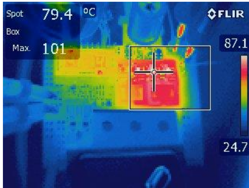
Figure 6.22 - Thermal Image of Limited Current on Controller 1
