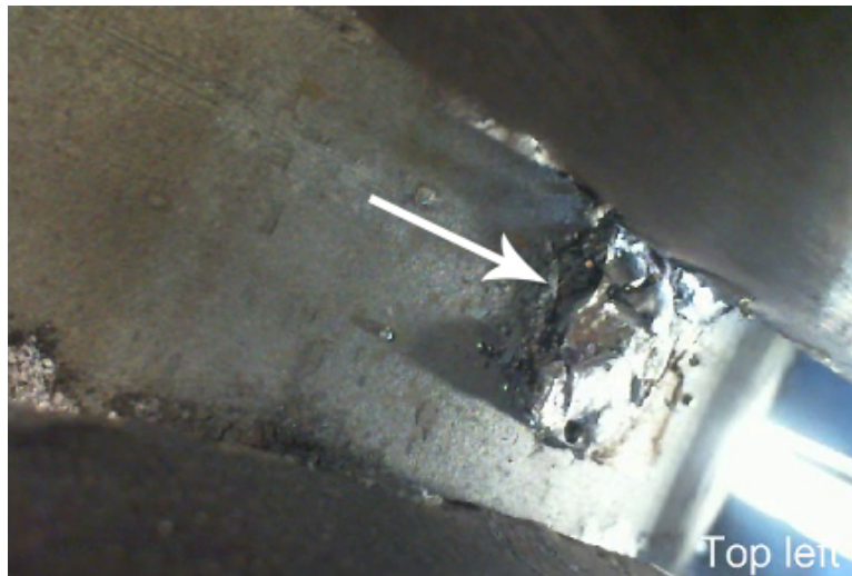
Figure 6.40. Fracture initiation under a puddle weld.
