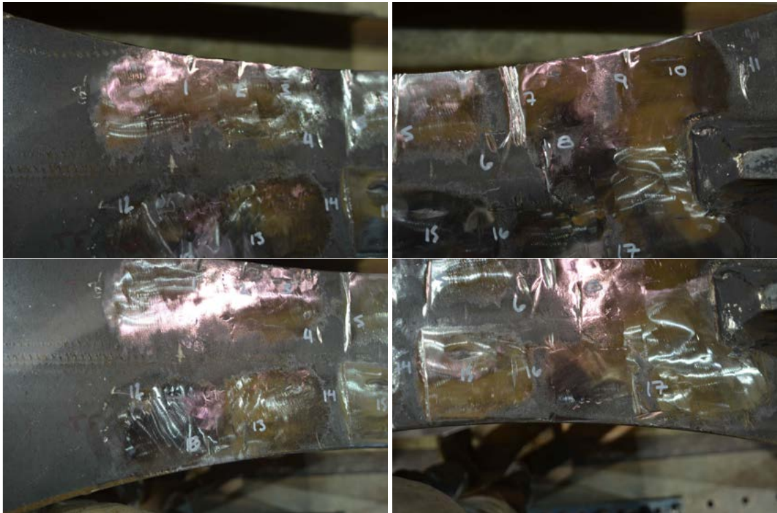
Figure S.6. Top flange defects.
