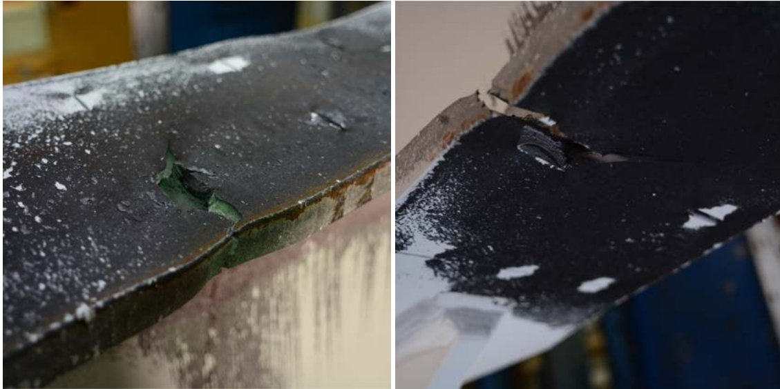
(a) Top flange fracture.
