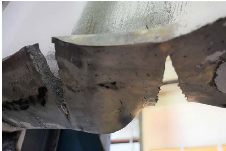
Figure 6.17. Bottom flange fractures on W36RBS-0.25NGTW-T94.
