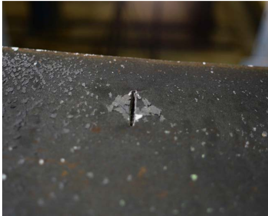
Figure 6.27. Fracture initiation in the bottom of notches on W36RBS-0.25N-T94.
