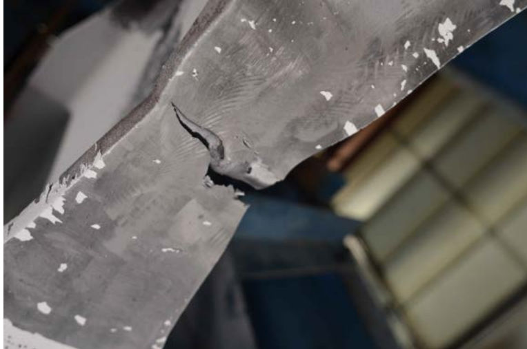
Figure 6.13. Bottom flange fracture of W24RBS-0.25NGTW-T59.
