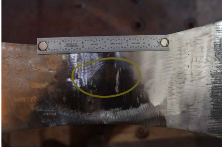
Figure S.4. Second top flange surface crack.
