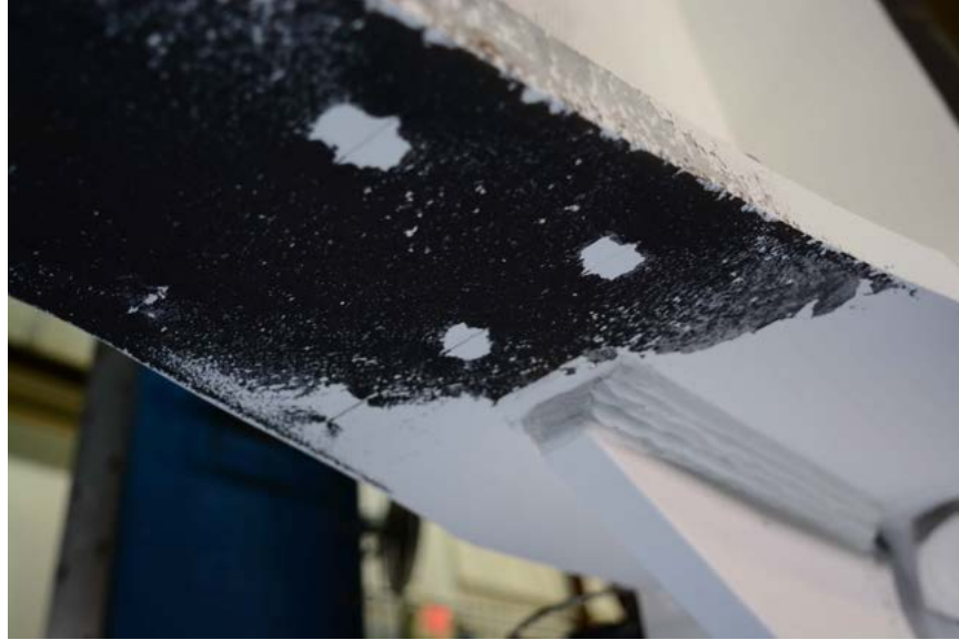
Figure 6.26. Notches closed up due to local buckling..
