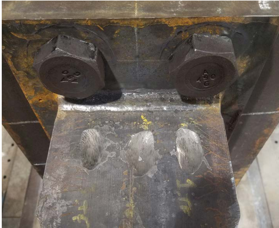
Figure 3.6. Finished 0.125 in. notches repair by grinding.
