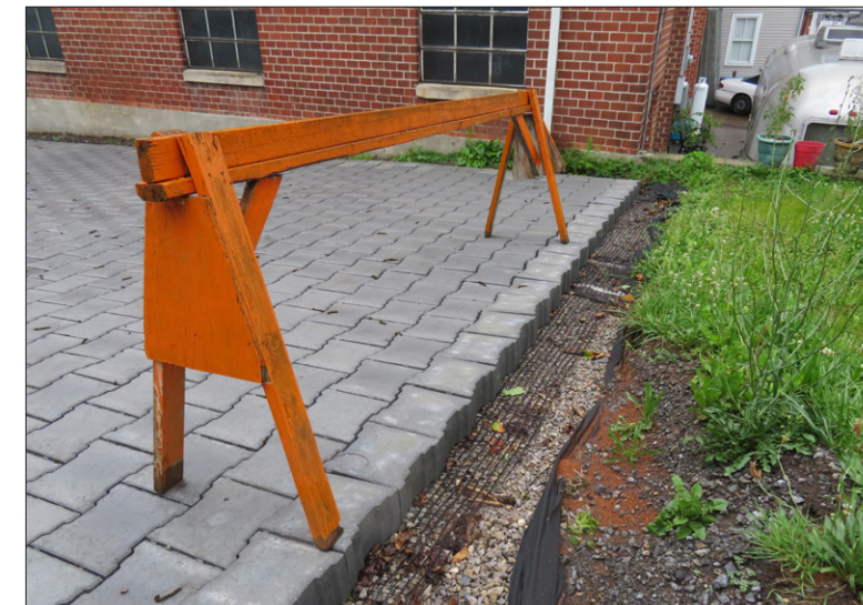
Permeable paving systems provide increased water retention during storm events and minimizes runoff to surrounding water ways.
