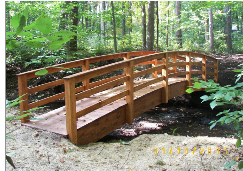
A pedestrian bridge creates access across Hawksbill Creek to connect the existing greenway into the new community space.
