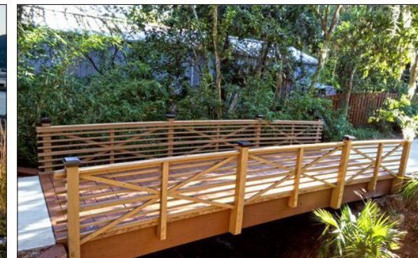
A pedestrian bridge creates access across Hawksbill Creek to connect the existing greenway into the new community space.
