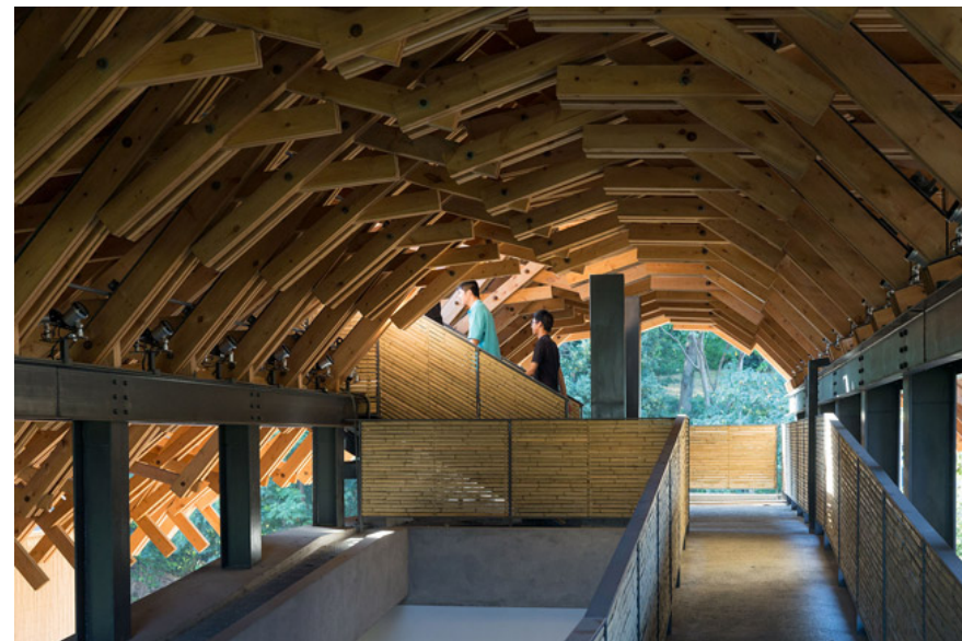
Exposed steel frame on top of the wall [6]
