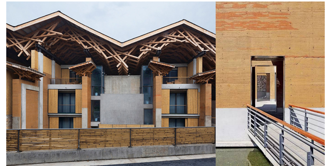
Concrete base and edge [6] [7]
