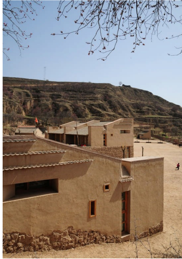
Classroom with shed roof [8]
