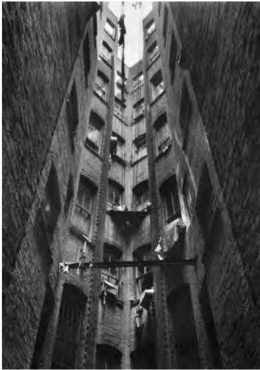
6.3. The tenement problem. The Dumbbell plan (6.3a, top) resulted in dingy, narrow airshafts (6.3b and 6.3.c, above) that were almost lightless and airless, though they were an improvement on older tenements.
