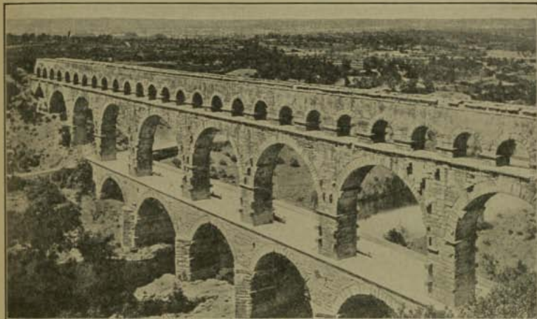
Ancient Aqueduct, Nimes, France
