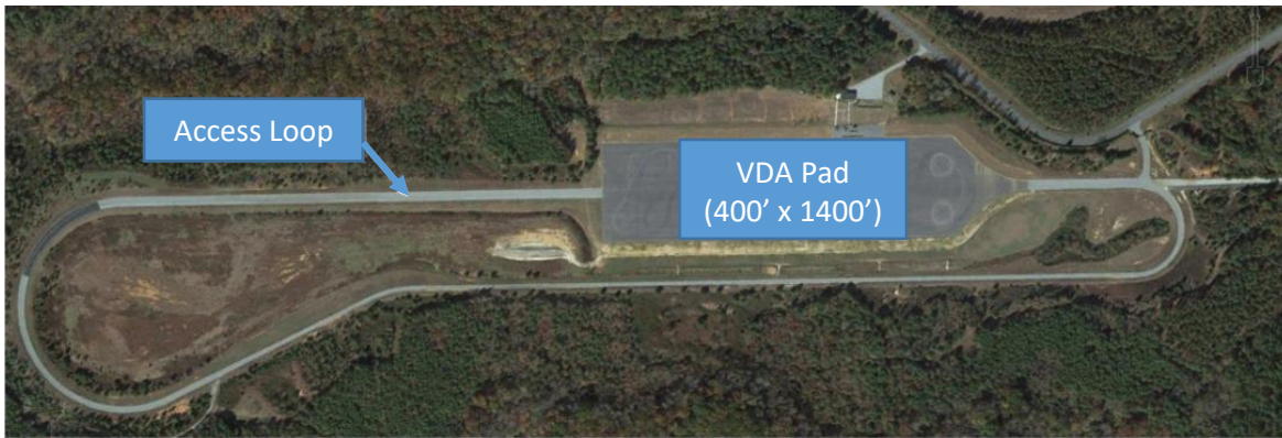
Figure 4-30. Track 8 at Michelin Laurens Proving Ground via Google Earth.
