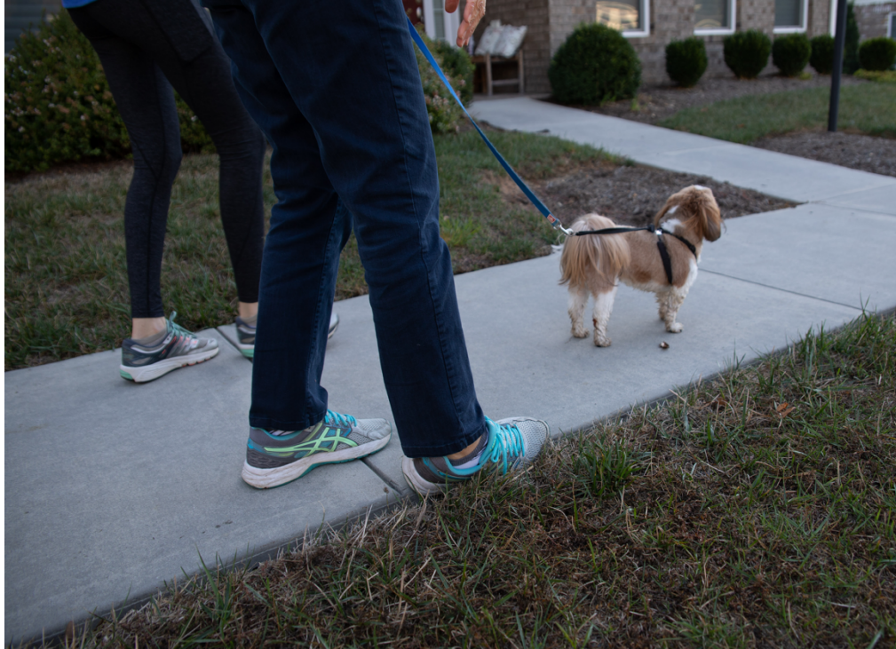
Figure 4.6. Tripping hazard along sidewalk where trench has formed
