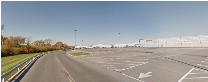
Image 43: Looking from the south western entrance
