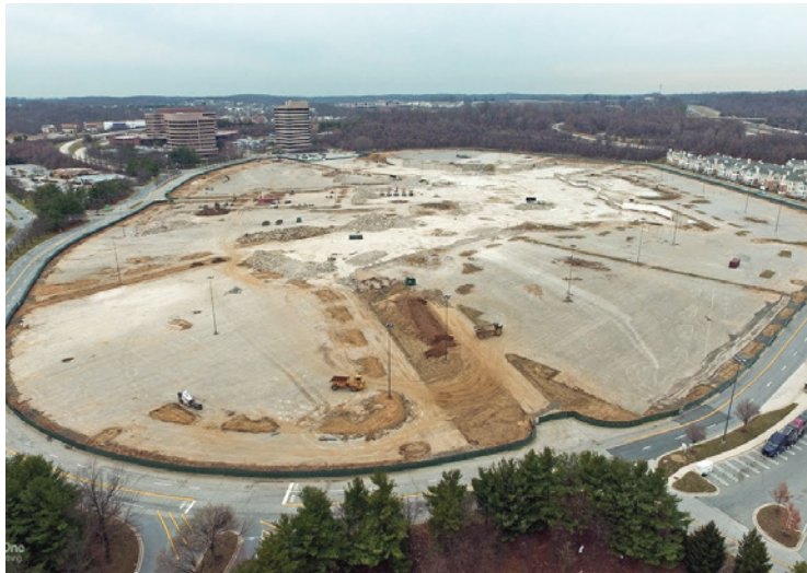
Figure 6: Aerial view of demolished Owing Mills mall in Baltimore, MD
