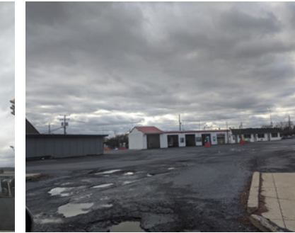
Image 46: Existing road condition
