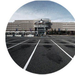
Figure 14: Asphalt parking lot at Mall of America, MN
