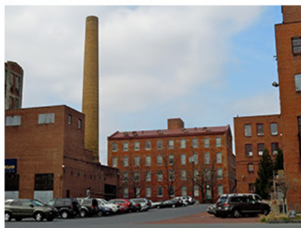
Reading Hardware Butt Works
