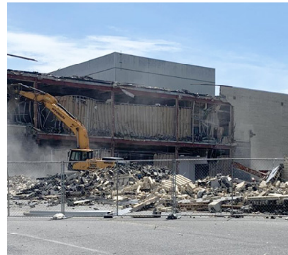
Figure 38: Mall being demolished, 2020
