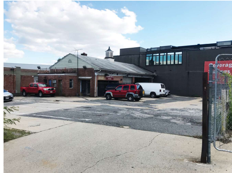
Existing Structure + Parking Lot - Looking SE
