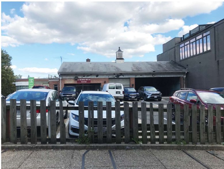
Existing Structure and Edge Condition - Looking East
