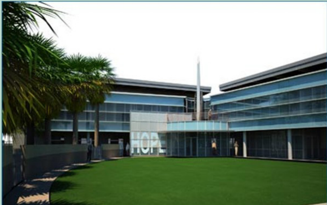
Fig. 47. (top) public facade; (bottom) private courtyard.
