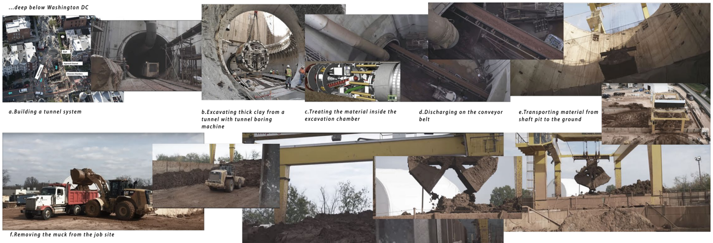
Figure 12. The Tunneling Process, Deep Below the Washington DC
