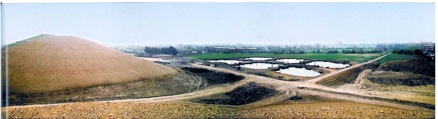
Figure 20. The Construction of the Mounds, Northala Fields Park
