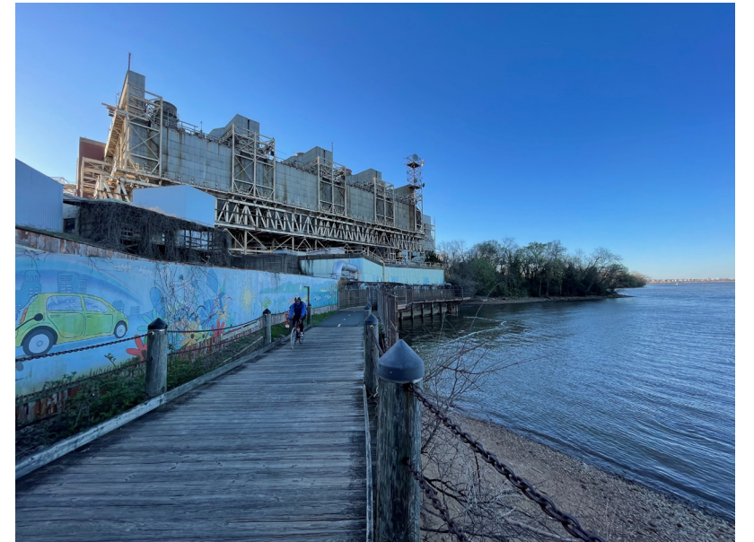
3 Alexandria Coal Power Plant
