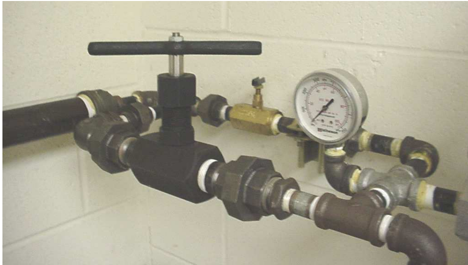
Figure 2.4: Flow rate regulating valves
