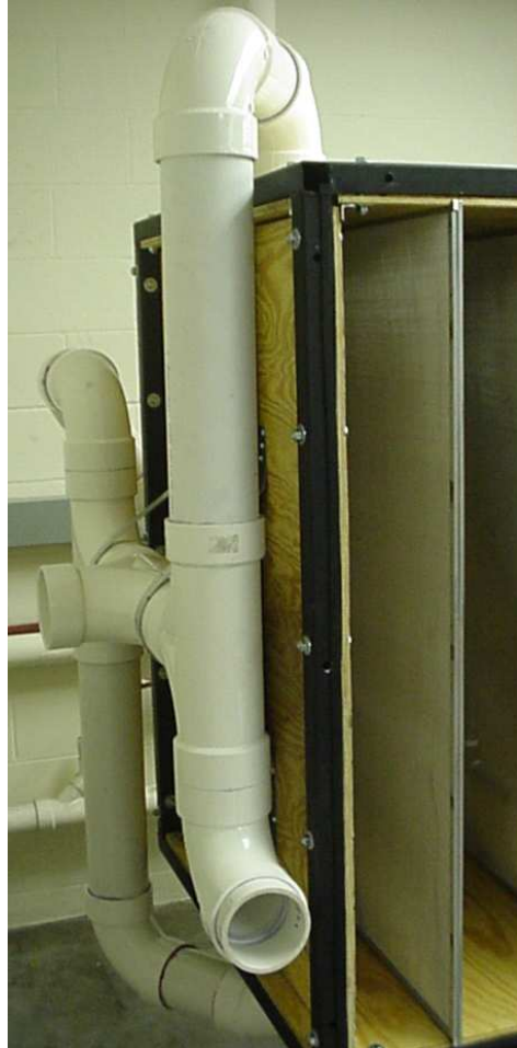
Figure 2.7: PVC pipe settling chamber inlet
