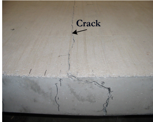
Fig. 3.4 Typical concrete cracking after failure
