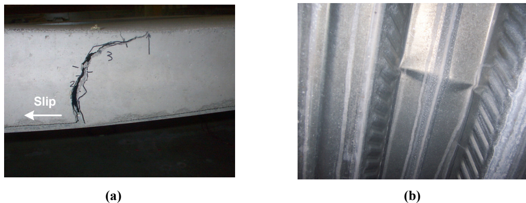
Fig. 3.3 Concrete cracking and flange buckling (a) Major crack due to slip failure. (b) Buckling of deck top flange
