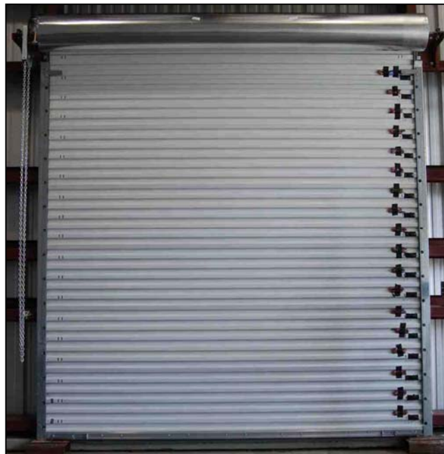
Figure 1. Steel curtain rolling sheet door (view from the inside of a building)
