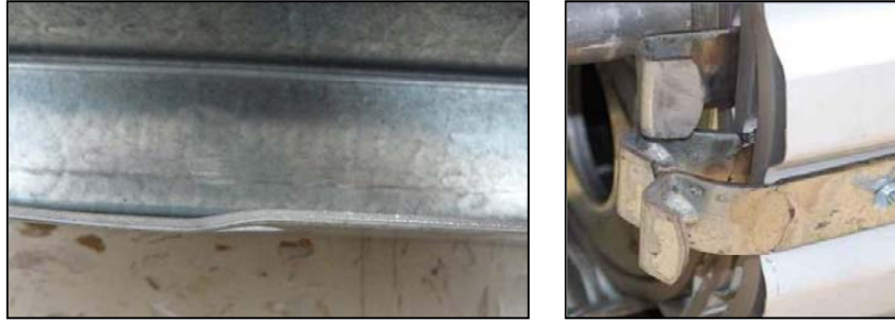
Figure 33. Bended wind lock and wind-guide after positive testing
