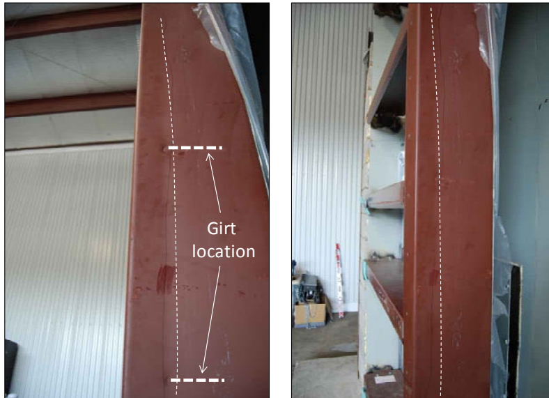
Figure 35. The web was plastically deformed at a seam corresponding to the welded girt connection plate
