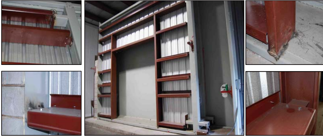
Figure 5. Door frame details (picture taken from the inside of the building)
