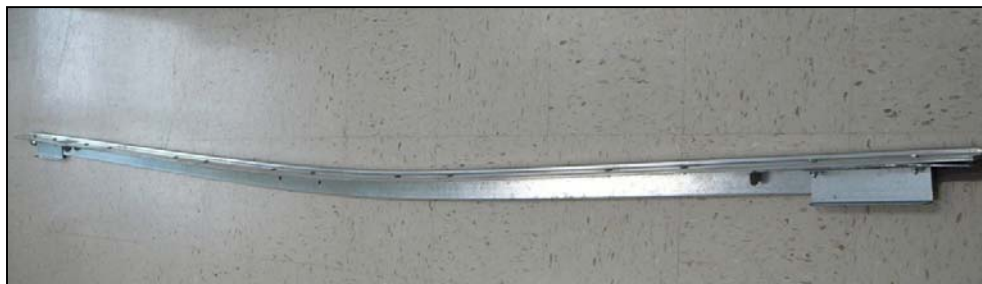
Figure 20. Bottom door angle was severely deformed after Door #1P-3 (+140 psf max)
