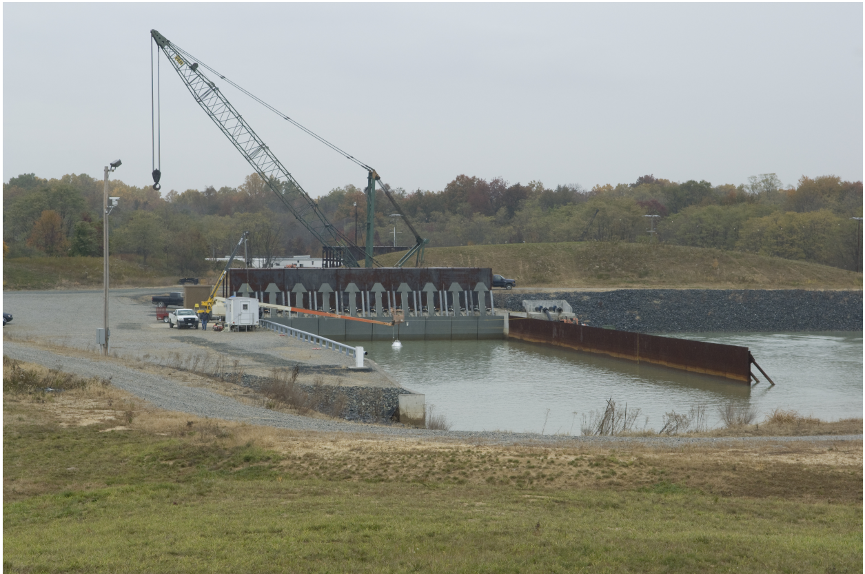
Figure 2.4: LWE with channel wall in place.[1] Photo used with permission.
