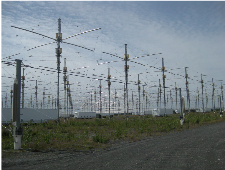
Figure 2.4: Photograph of the HAARP antenna array
