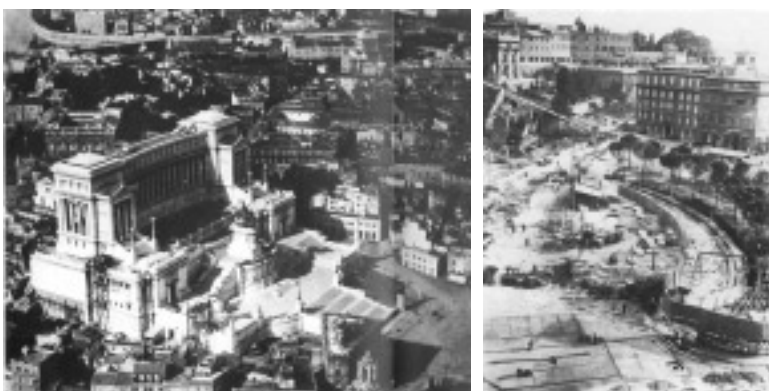
Figure 47 and 48 - View Looking Southwest to the Vittorio Emanuele II Monument during construction
