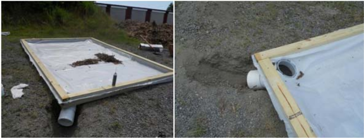
Figure 4. Plot 2: Impervious base (left) with drain for leachate collection at lower corner of plot (right). Drainage valve not shown on PVC elbow. Plot 2 and Plot 3 were constructed identically.
