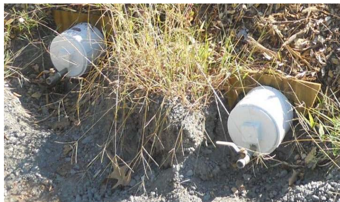
Figure 3. Plot 1: Drainage valves at lower end of lysimeters.
