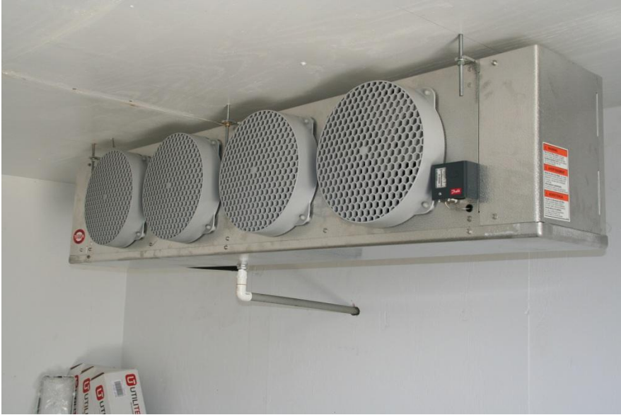
Figure 9. New Walk –In Cooler Chilling Capacity and Wall Insulation
