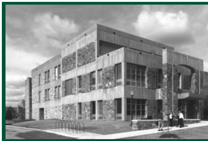
Julian Cheatham Hall - New Addition Completed 2003
