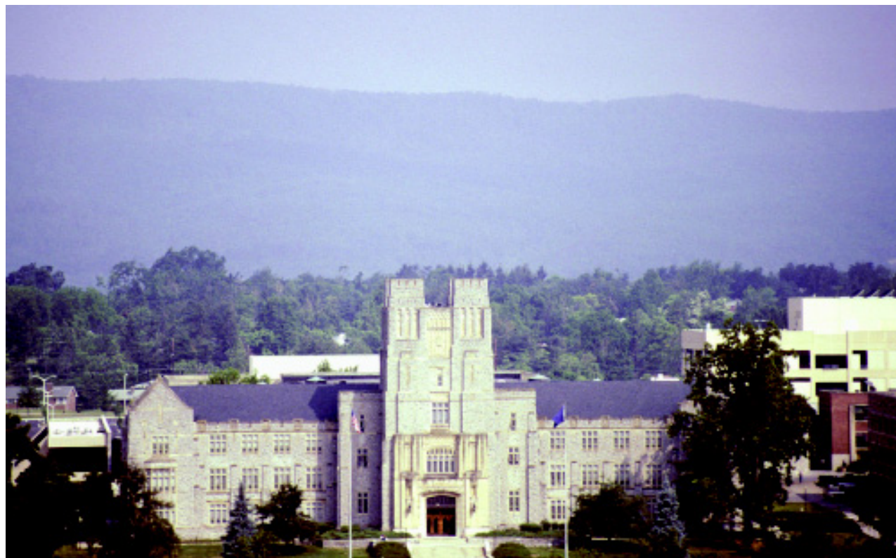
Aerial view of Burruss Hall, Virginia Tech campus.
