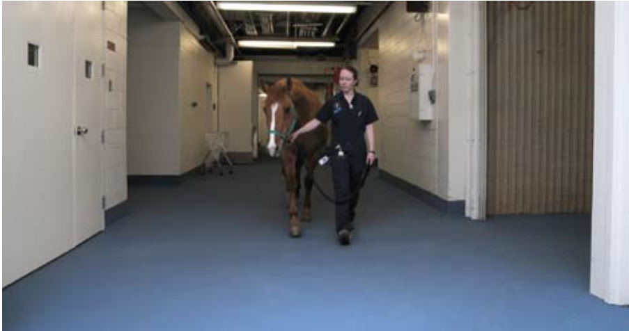
The Harry T. Peters, Jr. Large Animal Hospital has installed a new flooring system to promote biosecurity, safety, and efficiency.
