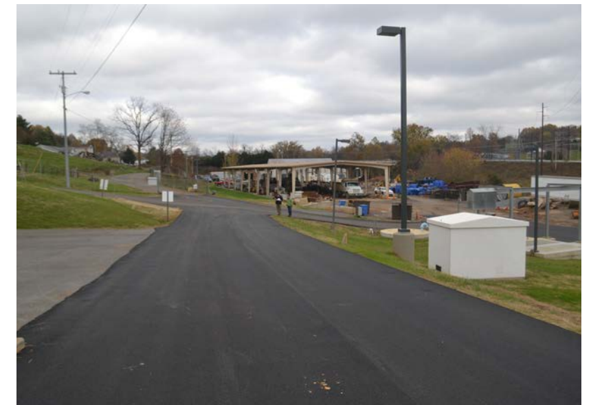
View looking North toward existing employee entrance on the upper site from the waste water treatment area.
