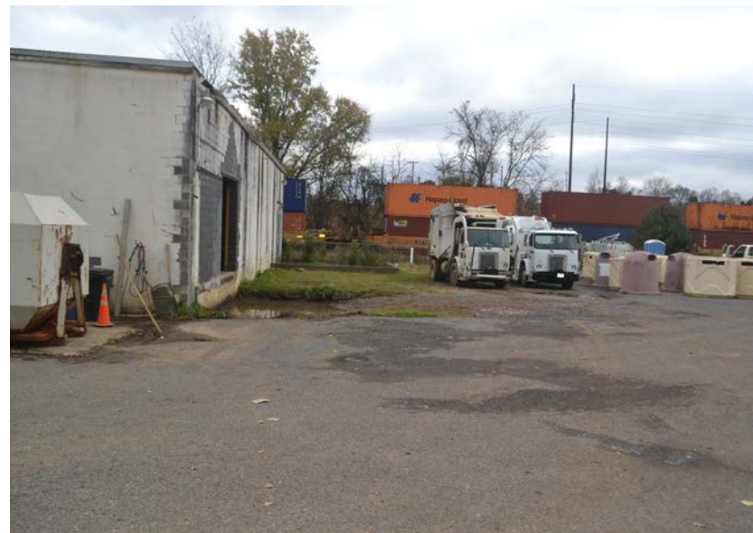
View of existing Solid Waste and Recycling building.
