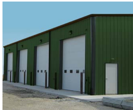
4. Storage structures painted green
