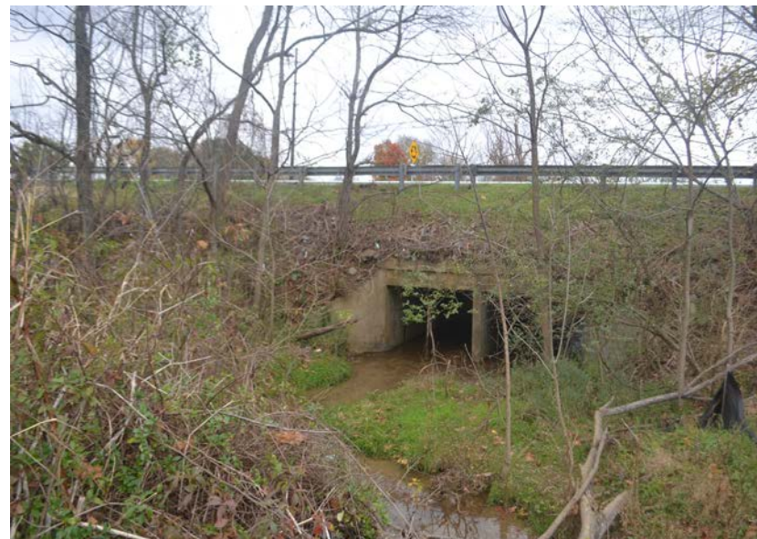
View of culvert under Main Street.
