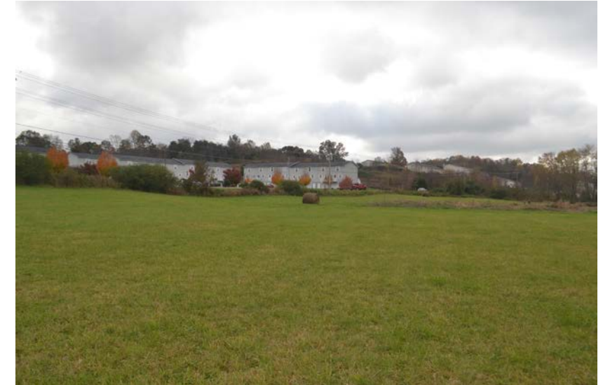
View looking South at an apartment complex from the Rosenbaum property.
