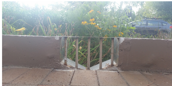
Runoff water is funneled into grates where it irrigates plants, cleans water, and returns water to the ground, keeping it out of the sewer.
