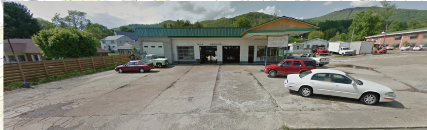
Existing Conditions: A view northward at the corner of West Main Street and Hillside Drive at this auto garage is an example of a large building setback with an expansive concrete building front condition. This provides no street corridor enclosure and is an uncomfortable setting for pedestrians.
