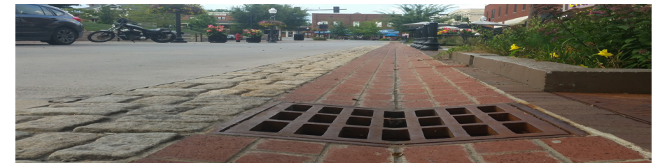
An alternative to traditional curb and gutter, street runoff water is diverted into brick channels and into drain inlets. Stone paving acts as a rumble strip and keeps cars from drifting into the sidewalk.
