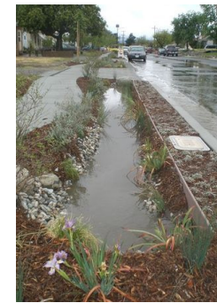
Example: In a large rain event, water is concentrated in areas where it can be returned to the groundwater supply
