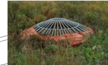
Example: Wetland overflow drain
