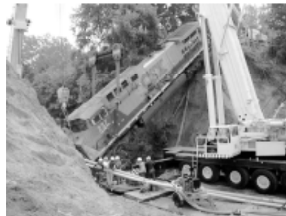
Figure 2: Flooding has caused significant property damage throughout Mecklenburg County. In this photo, a CSX railroad engine is pulled from Little Sugar Creek after floodwaters washed out the railroad bridge supports.
