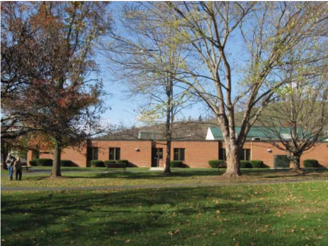
View of Meadowbrook Center courtyard.
