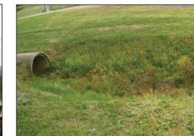
5. Drainage pipe and stream
