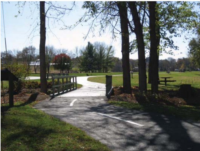
Pedestrian bridge on the Luray Hawksbill Greenway.
