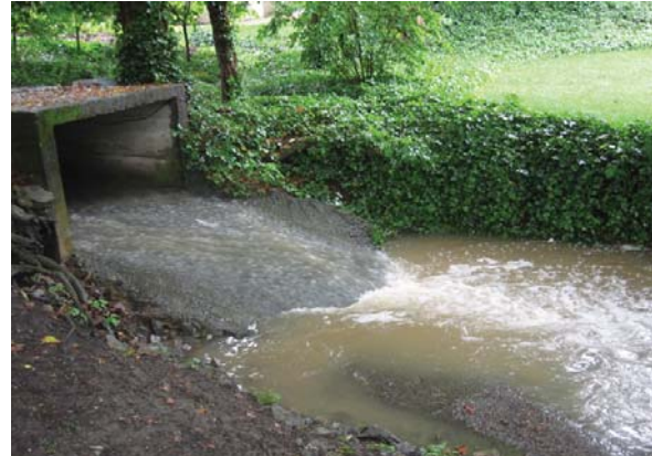
Inlet structure into the Five Chimneys site (Figure 1)
