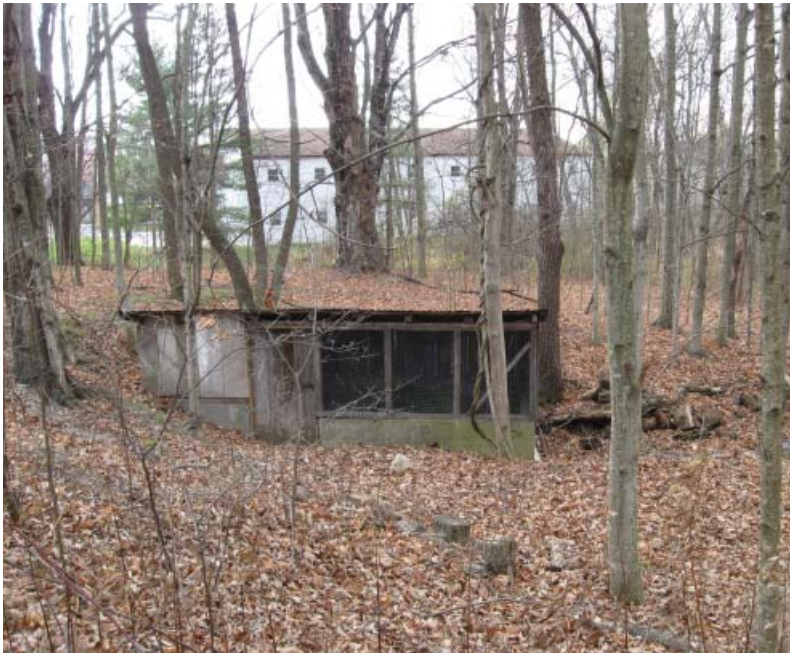
View from outside of the spring house
