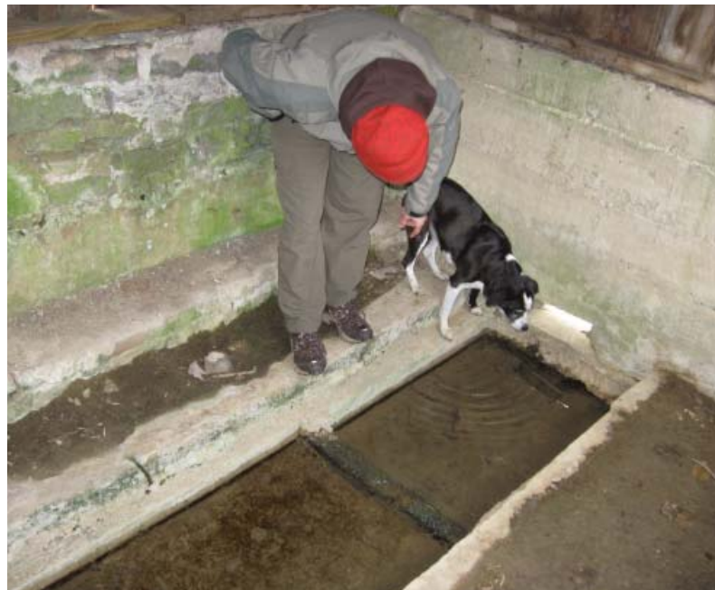
Inside a spring house that also feeds into Stroubles Creek
