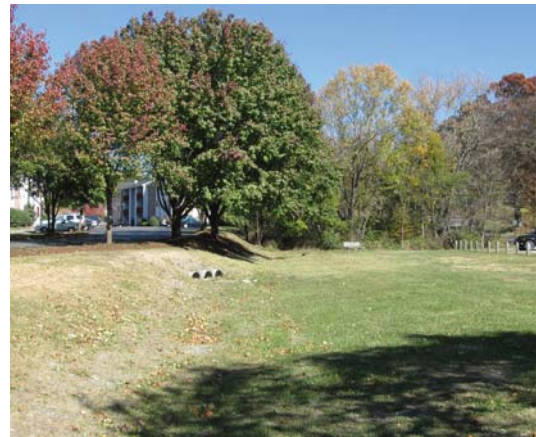
Initial site photo at Spout Spring Park
