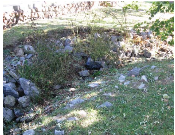
Eroded streambanks throughout the site (Figure 2)
