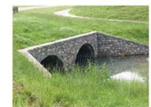
In order to approve the aesthetic qualities of the site, refacing the inlet structure with stone will improve its overall appearance.
