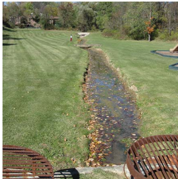
Owens Street Park above outlet structures (Figure 2)
