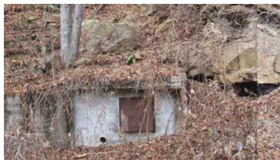
A mine portal with exposed coal seam immediately to the right.
