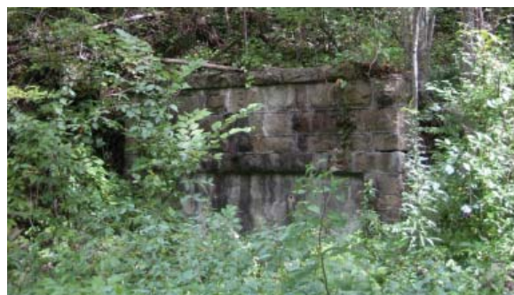
A sealed mine portal along the primary section of proposed trail.
