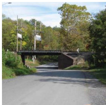
Train Trestle on Luray Avenue.
