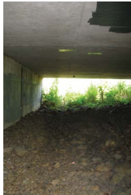
Area beneath the South Street Bridge.
