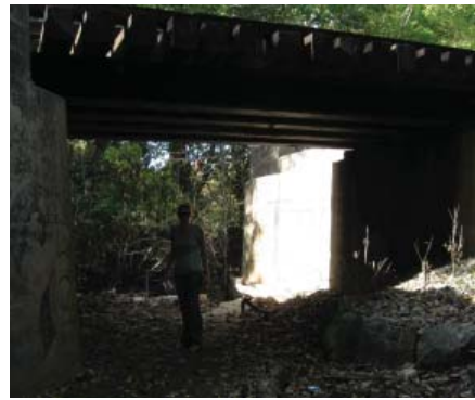
Eliza Furedy provides a scale to the culvert under the railroad tracks.
