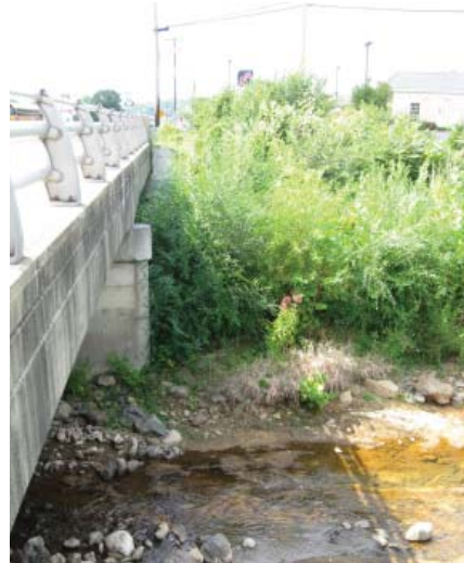
South Street Bridge
