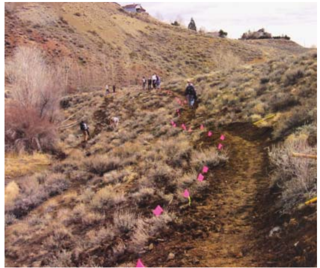
Example of digging the tread
