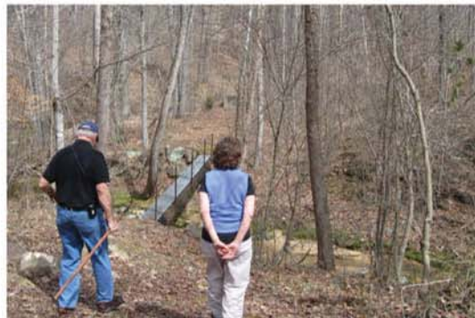
9. Sewer line and stream
