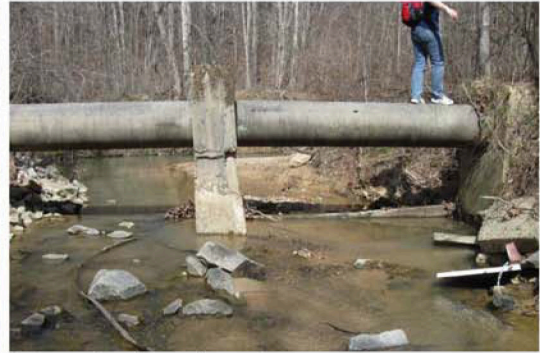
4. Sewer line above the creek
