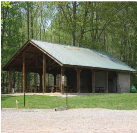
Example image of covered shelter with storage.
