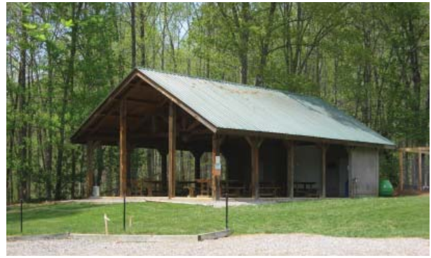
Example image of covered shelter with storage.
