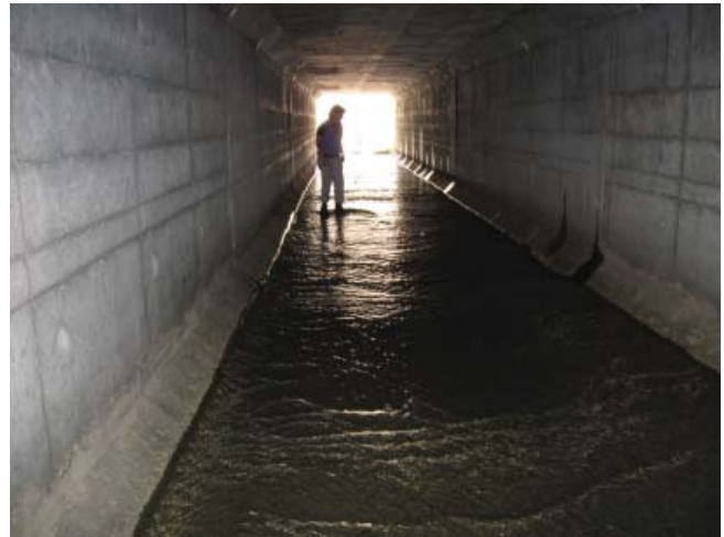
A CDAC project team member explores the existing box culvert under US 29 as a possible pedestrian connection between Zones 1 and 1 of the site.
