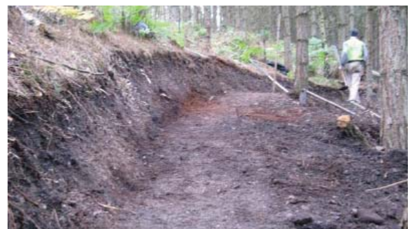
Example of finished backslope
