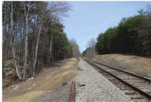
2. Railroad (facing northeast)
