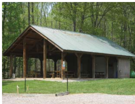
Example image of covered shelter with storage.
