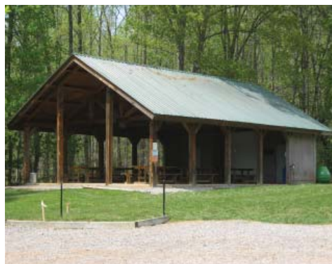
Example image of covered shelter with storage.
