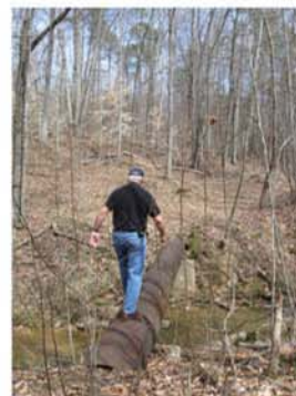
11. Sewer line above stream
