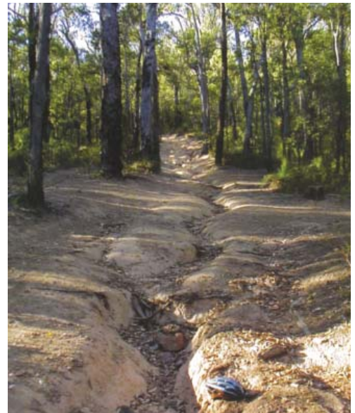
Example of erosion caused by a trail sited straight downhill
