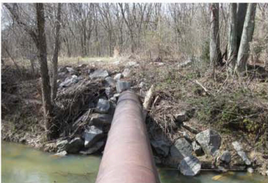
6. Sewer line across the Fall Creek
