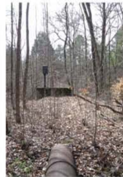
12. Sewer line underground
