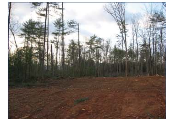
Post-tree harvesting next to existing parking lot
