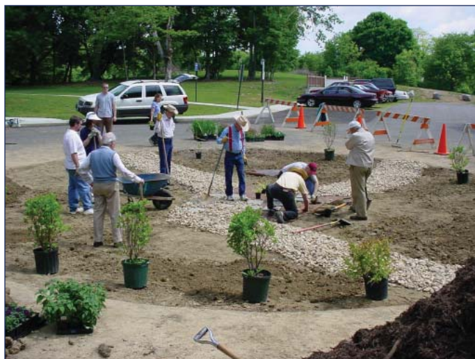
A rain garden under construction
