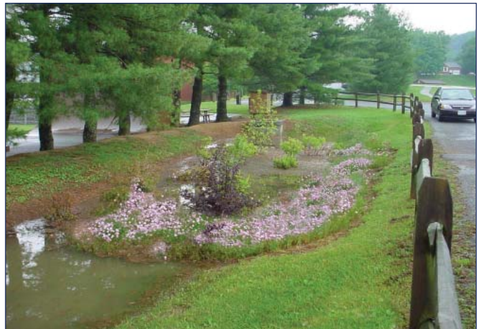
This garden, under construction in the picture above, is now planted and hard at work.
