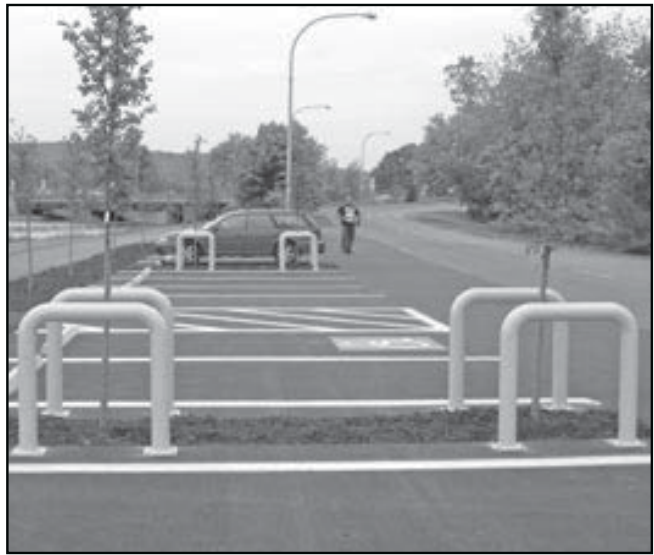
Here is the Ithaca, NY parking lot in the first year after planting. 'Accolade' elms were planted in the porous asphalt and traditional asphalt. Both surfaces have CU-Structural Soil underneath. We will be evaluating the growth of all trees in both surfaces over time.
