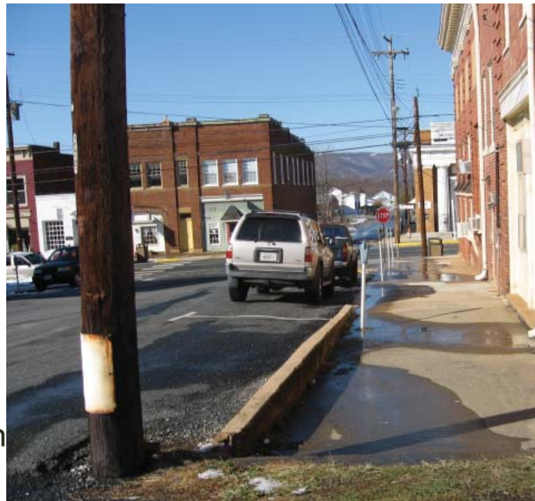
Sidewalk with an unusual curb situation, along with runoff problems. The sidewalk terminates into the grass along an access road.
