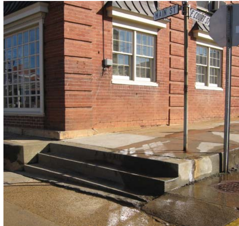
Walkway along East Court Street. Stairs added to deal with the steep slope, making the curb higher than average.
