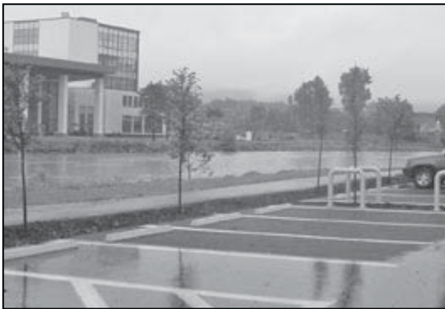
This is a 14-car parking lot in the city of Ithaca entirely built on 24" of CU-Structural Soil. In this rainy picture you can clearly see the traditional asphalt as it looks slick from the water running off it compared with the porous asphalt, which looks dull as rainwater goes through its surface. Subsequent to this construction, areas of both types of asphalt were cut out and elm trees were planted.
