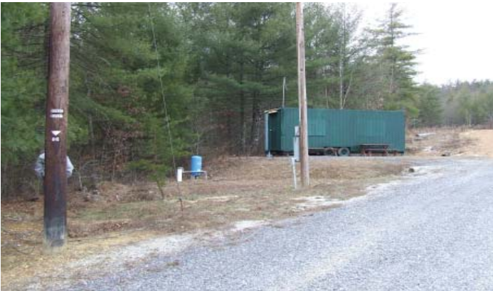
3. Existing access road and concession stand at the Col. Tom Dotson Sports Complex .
