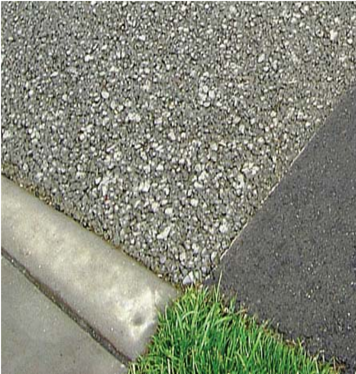
Photo of porous pavement. Photo taken from www.concretenetwork.com
