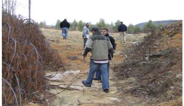
4. Depressed and eroded area at the edge of the Col. Tom Dotson Complex.
