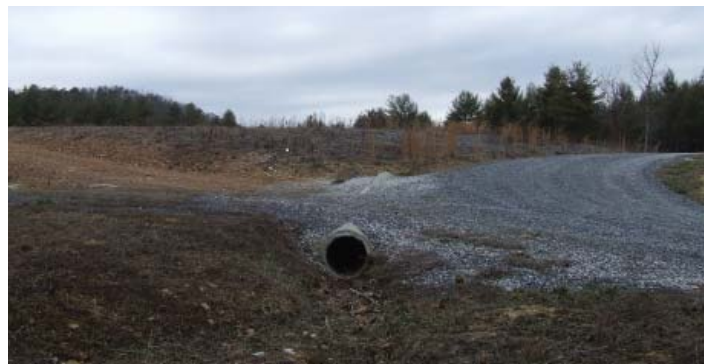
Existing culvert and drainage swale installed to move storm water from the Col. Tom Dotson Sports Complex into the existing detention pond.
