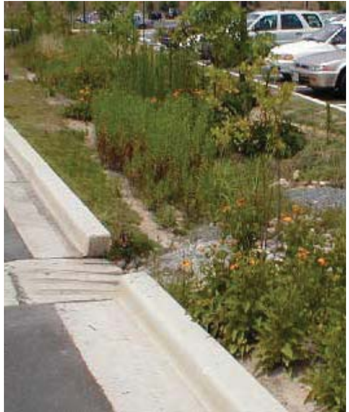
Example photo of a bio-retention parking lot swale. Photo taken from www.waterresearch.com
