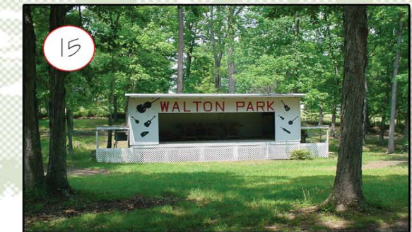
Performance stage affords great opportunities (needs general repairs)
