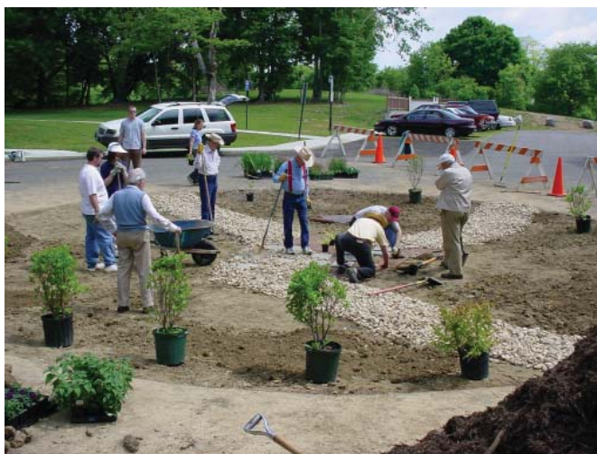
A rain garden under construction
