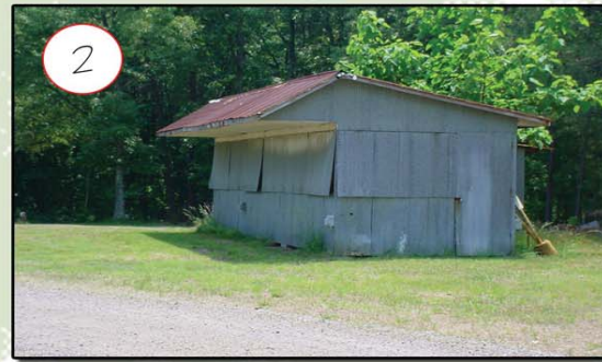
Storage structure in need of repair
