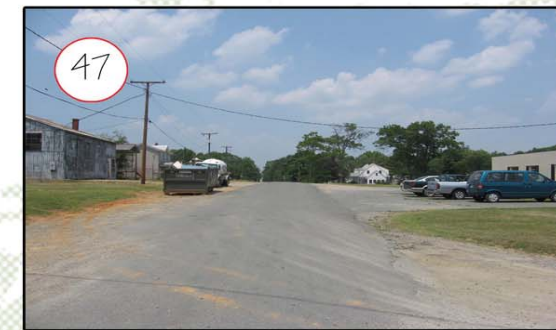
47 Site entrance road (poor quality) lacks directional signage
