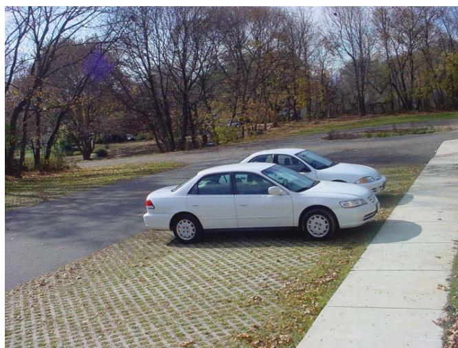
Porous pavers are used in the parking spaces while asphalt is used for the roadway surfacing.
