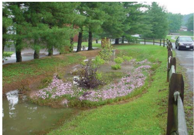
This garden, under construction in the picture above, is now planted and hard at work.
