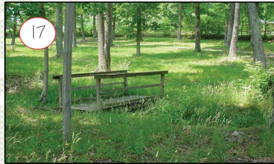
Unnecessary bridge structure
