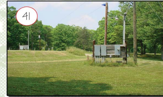
41 Unaesthetic quality of utilities
