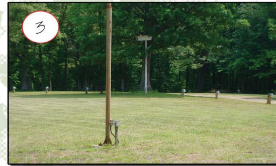
Flat open space: shows exposed utilities that may be screened and/or upgraded
