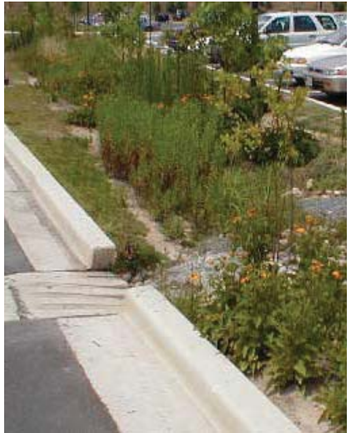
Example photo of a bio-retention parking lot swale. Photo taken from www.waterresearch.com
