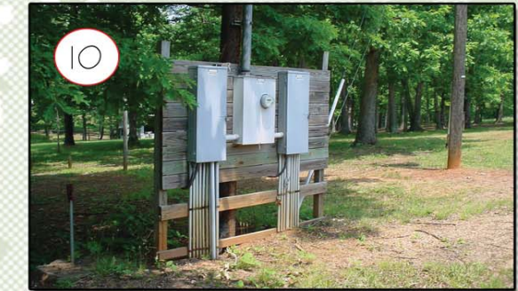
Exposed utility junction (unappealing)
