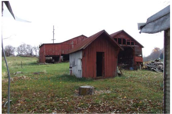
Condition of property outbuildings
