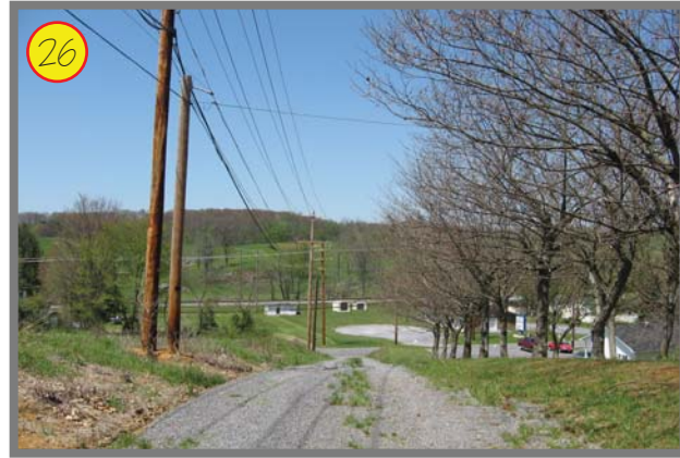
AEP station access road quality: substantial upgrade needed
