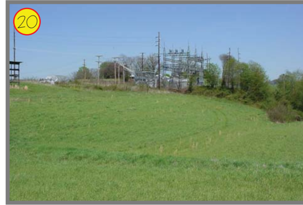
AEP Station with tire tracks indicating AEP access from onsite
