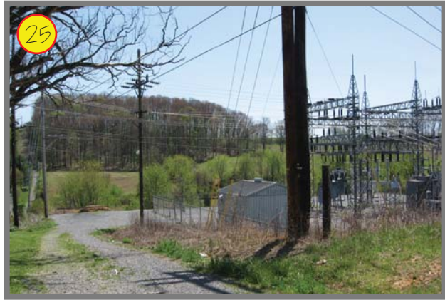
View of AEP station: possible site access point
