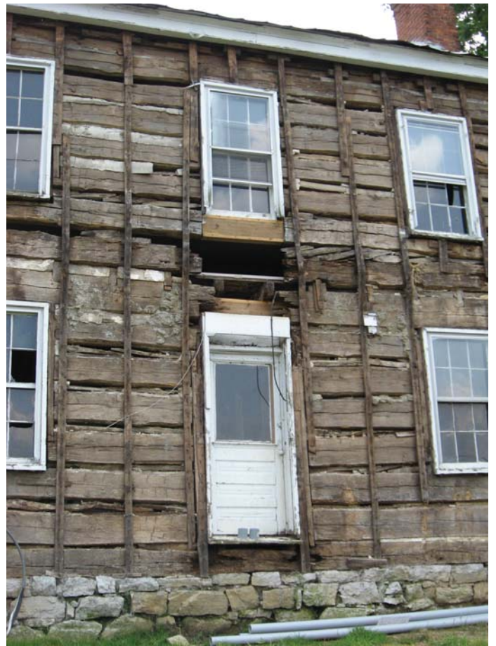
Close-up view of the logs used in the construction of the Hagey house.
