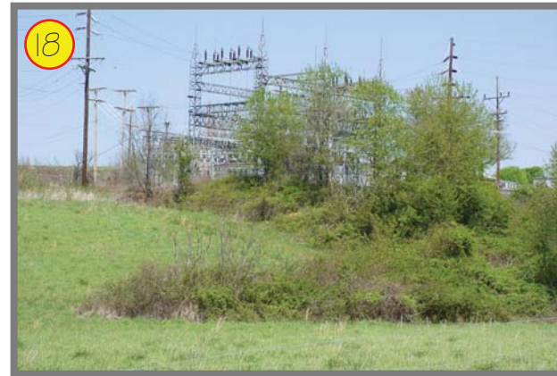
Unappealing view of AEP Station
