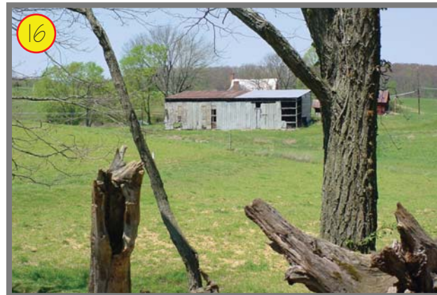
Slightly obstructed view of barn structures
