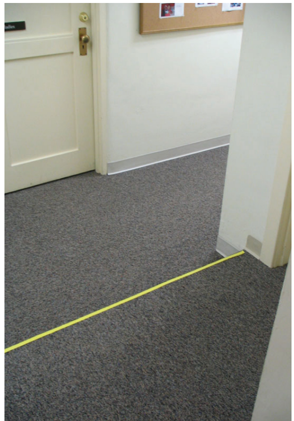
One of a number of level changes in the floor at the basement level is marked with a yellow line for safety.
