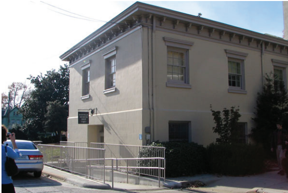
Rear accessible entrance to the basement level through the gift shop.
