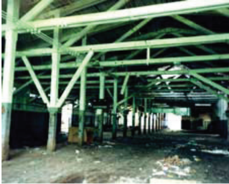
The interiors of mills and industrial buildings are frequently open, unadorned spaces with exposed structural elements. While these spaces can serve many new uses, the floor to ceiling height and exposed truss system are character-defining features that should be retained in rehabilitation. Photo: NPS files.
