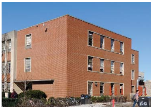
MSE now occupies labs and offices on the first floor of Randolph Hall on the east side and along the front of the building facing Holden Hall.
