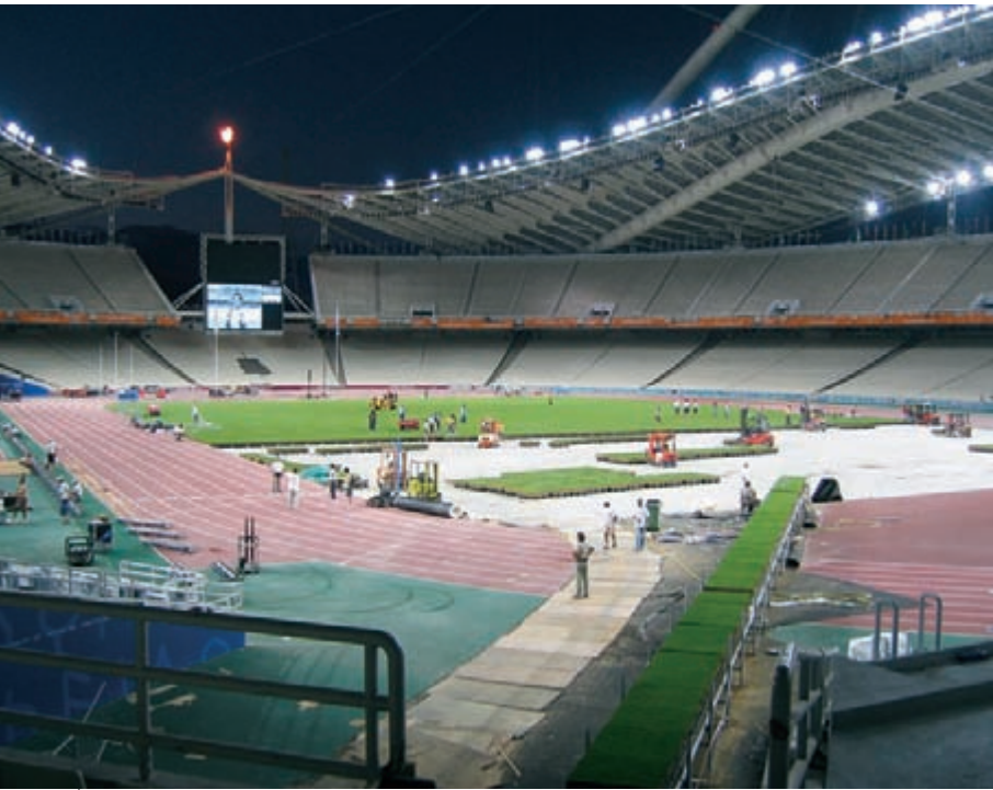
Installation of GreenTech turf at the Olympic stadium in Athens.
