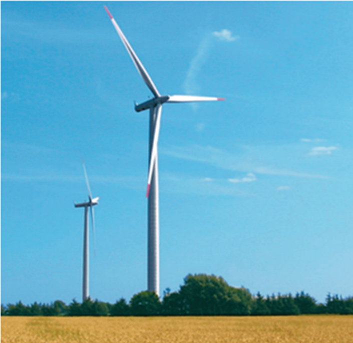
Figure 5 Siemens HAWT (model: SWT-2.3-82 VS) ( http://www.energy.siemens.com/us/pool/hq/power-generation/wind-power/E50001-W310-A123-X-4A00_WS_SWT-2.3-82%20VS_US.pdf )
