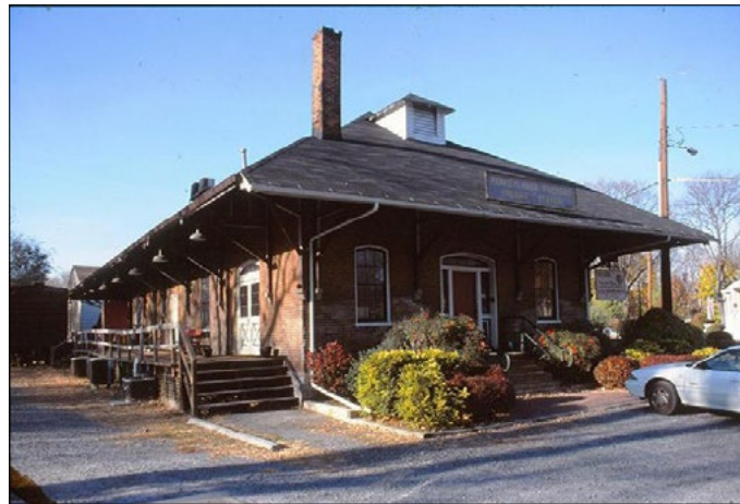
Original platform and stairs adjacent to tracks
