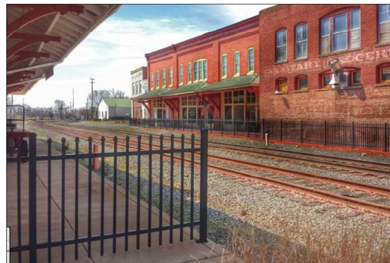
Lack of safety fence; required in Dante by CSX Railroad
