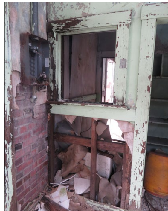
Interior ticket window
