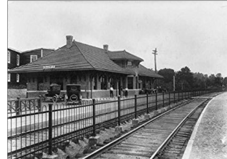
Historical image, 1920, and original railing style
