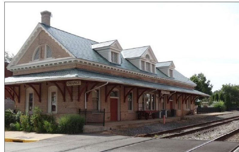
Depot adjacent to railroad tracks without safety fencing
