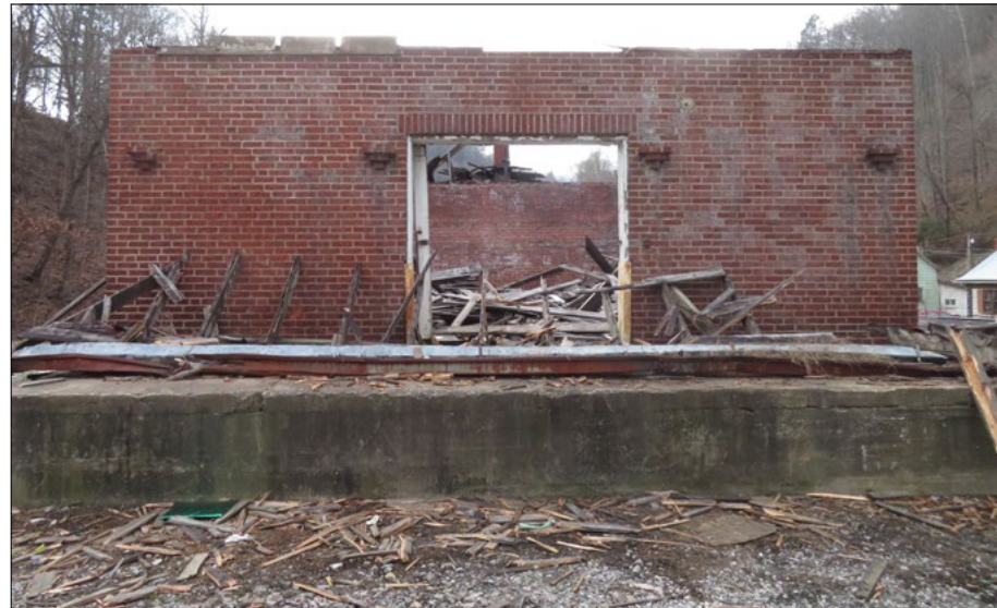
Northeast facade and existing train platform
