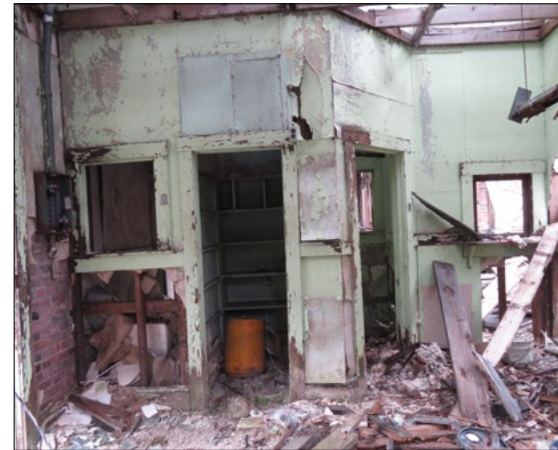
Former restroom and ticket window facing west
