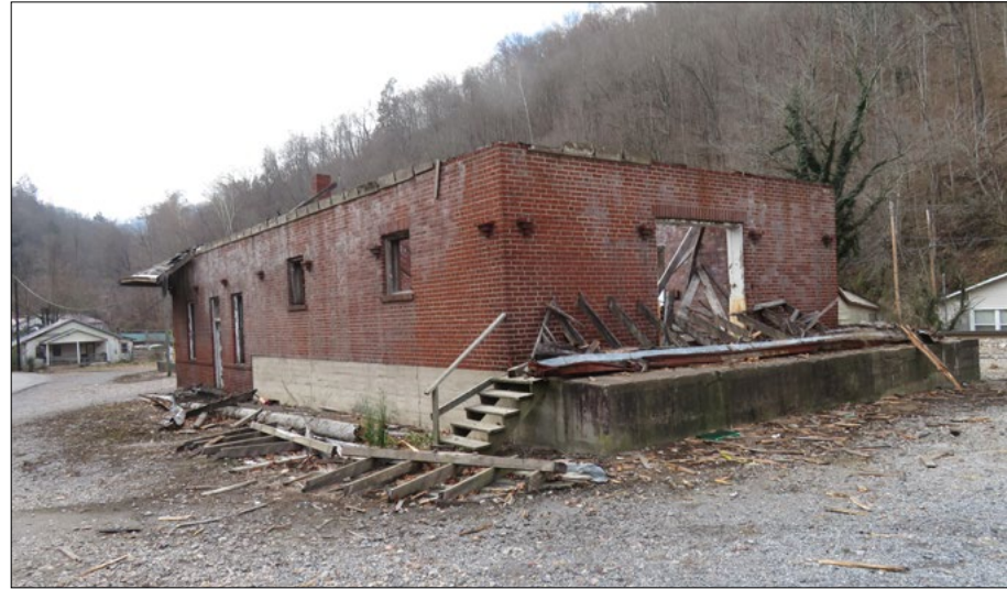
Northeast corner and existing train platform
