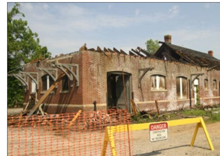
Pre-renovation with collapsed roof
