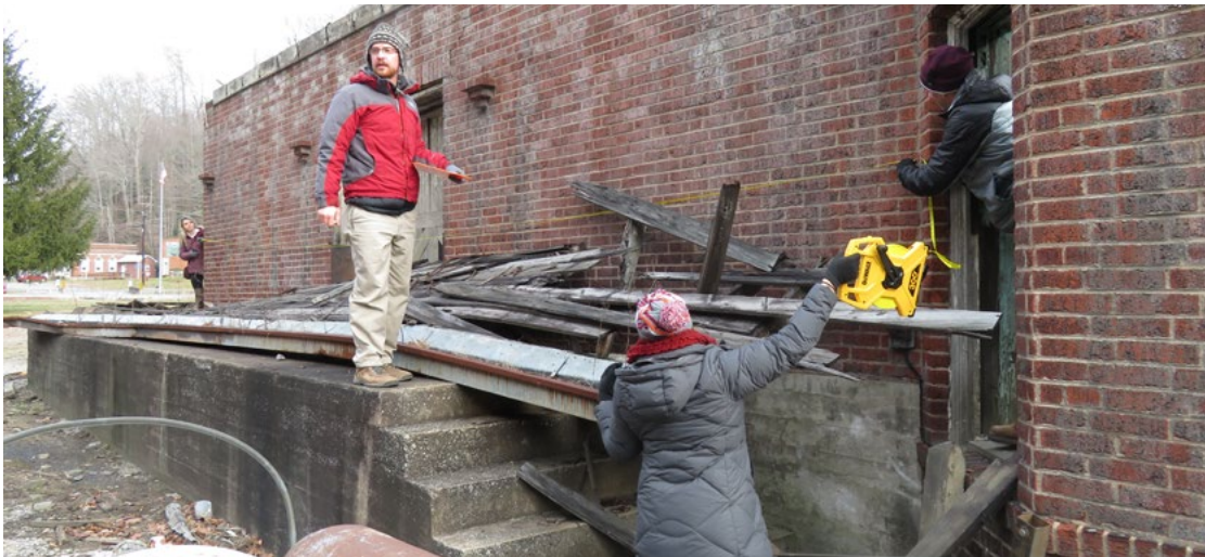
CDAC project manager Nick Proctor works with student designers Samantha Piotrowski and Meredith Tobias and Joe Morici of Cardno to measure the exterior of the Dante Depot.
