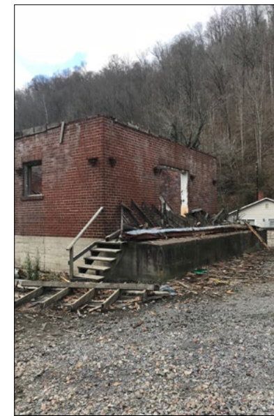
Northeast steps & platform
