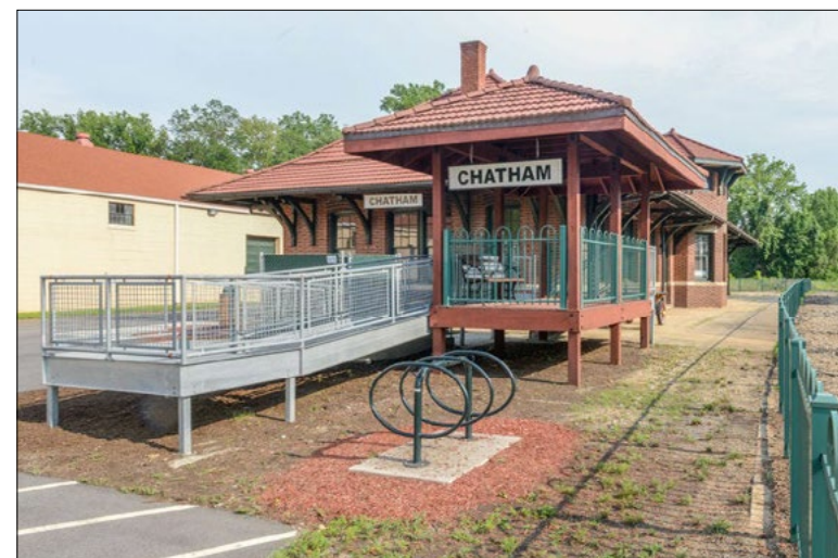
Modern ADA ramp railing does not match other fencing styles used around the structure
