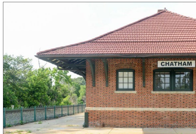
Renovated exterior with new signage, roof, and supports
