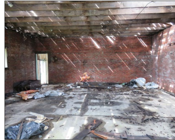
Interior view from northeast side
