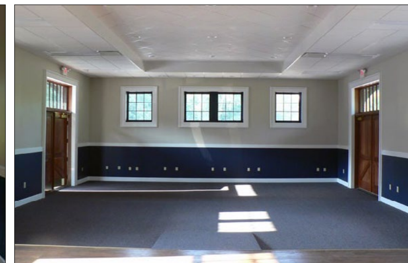
Interior view; variety of outlet placements and dropped ceiling
