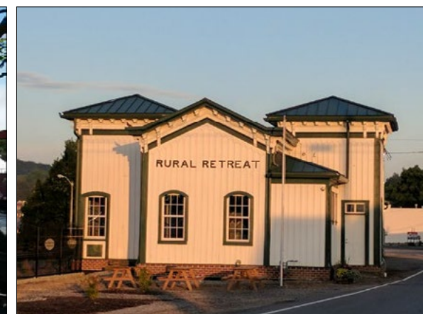
Renovated exterior featuring picnic tables and flag pole
