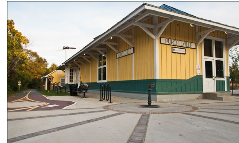
Additional amenities: bicycle racks, water fountain, and benches
