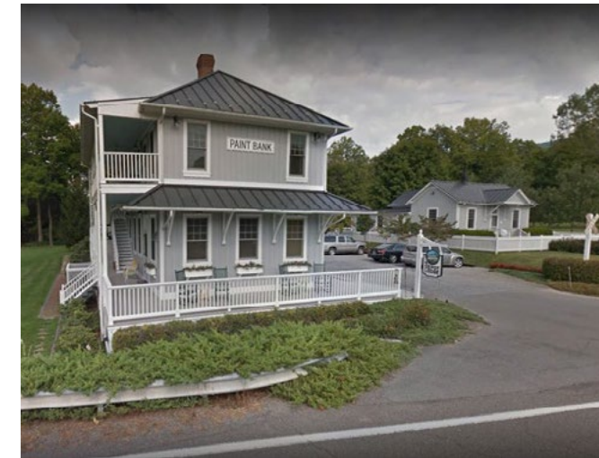
Depot Lodge (left) adjacent to surrounding houses (right)
