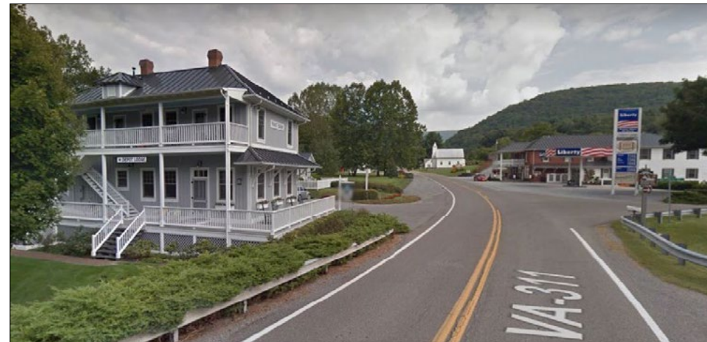
Architecturally unique from other depots due to the porches and multiple levels. Lodge view (left) as seen from VA-311
